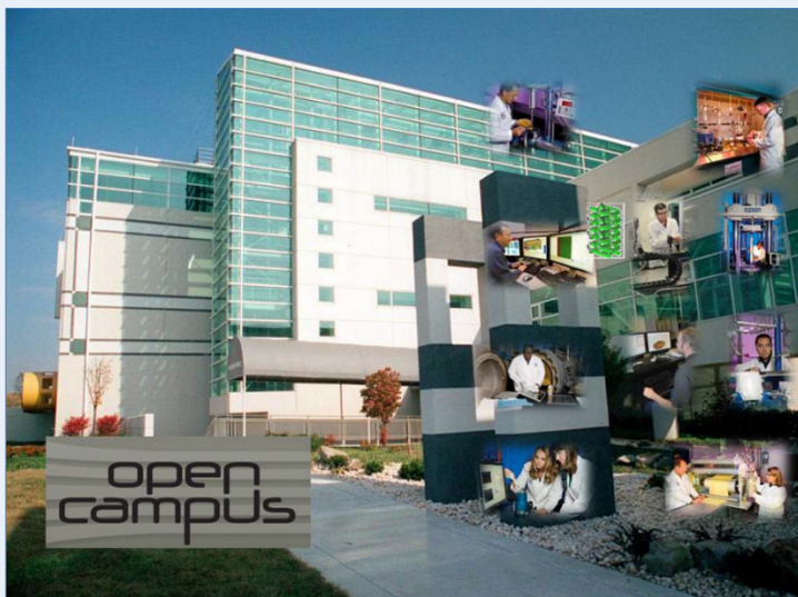
The Rodman Materials Research Laboratory, Aberdeen Proving Ground, Maryland. The Rodman Building is home to the U.S. Army Research Laboratory's structural materials research, and has extensive materials characterization and synthesis facilities for metals, ceramics, polymers, glasses, and composites. By utilizing the Open Campus framework, visiting scientists can work side-by-side with ARL scientists and engineers in ARL facilities such as the Rodman Laboratory. Find out more about Open Campus and other ARL facilities across the nation at www.arl.army.mil/opencampus/ .
